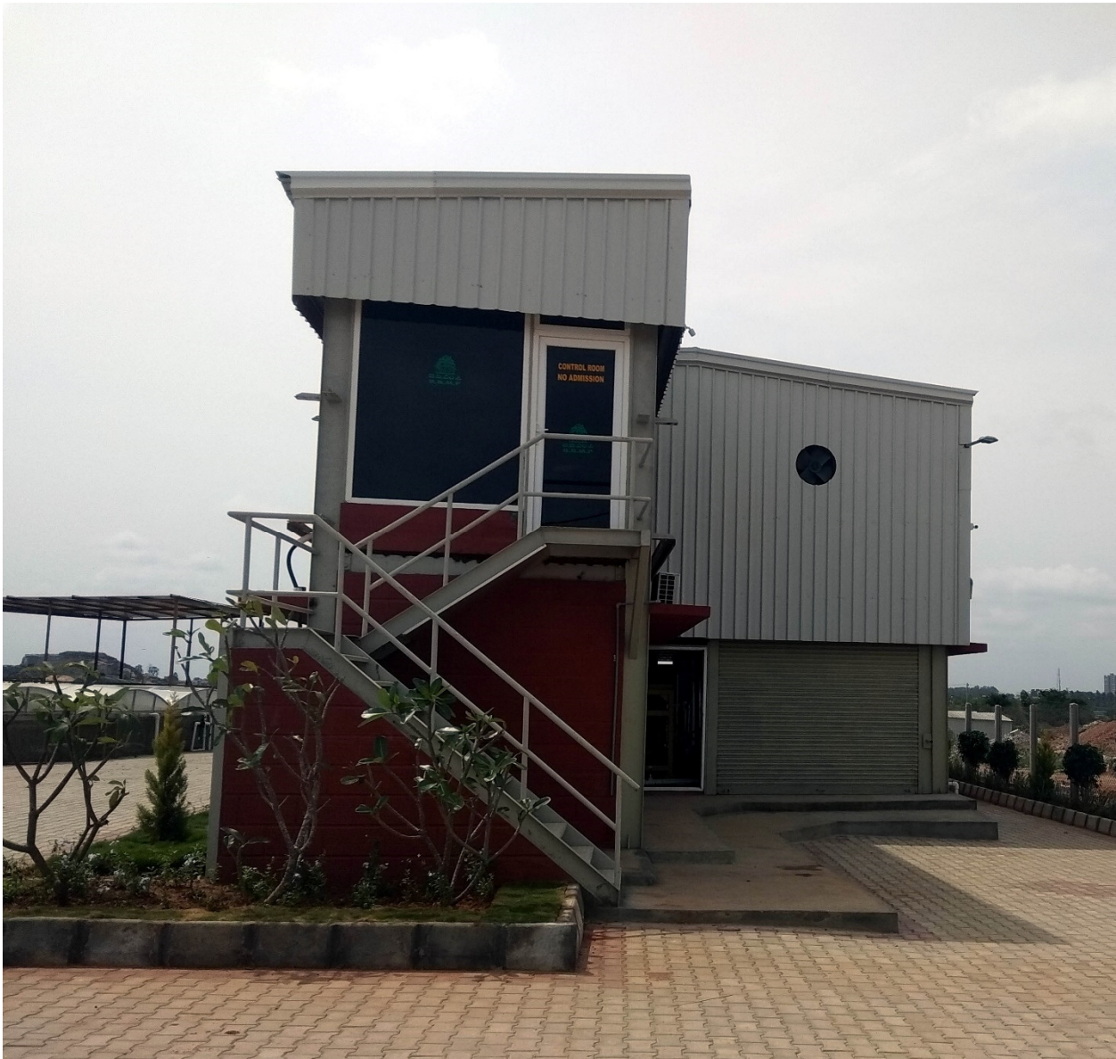
The State-of-the-art 120m 3 /day ZLD Landfill Leachate Treatment Plant at BBMP Landfill, Bellahalli, Bengaluru
